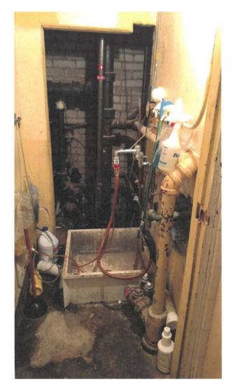
• The original domestic water piping is primarily galvanized that is in poor condition. Replace with new copper piping throughout. The 2005 Addition piping is in satisfactory condition.
