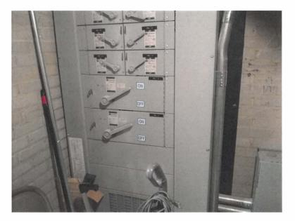
There is an old 800 amp switchboard that is beyond its useful life and should be replaced as a part of the electrical service upgrade. A number of old/damaged panelboards in the building are also in need of replacement.
