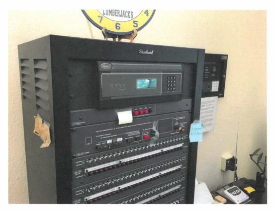
The existing clocks are a mixture of digital clocks in the corridors and non-synchronous clocks in the classrooms and miscellaneous spaces. For overall better performance, it is recommended that a new, synchronous clock system be installed across the Junior High and High School.
