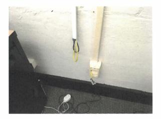
The existing AV cabling in the classrooms is analog VGA type. As the classroom projectors are replaced (currently about 50% of the projectors are replaced) along with new computer updates for staff, only an HDMI cabling solution will work.
