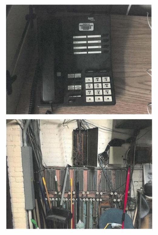
• The data cabling in the building is currently a mixture of Category 5, 5E and 6. There are locations in the building where the cabling is damaged. The type of cabling needed to increase the speed of the overall system to an effective 10Gb and the bandwidth is 6A. This upgrade includes cabling to faceplate connections and the wireless access points. Additional wireless devices will be able to access the network at an increased speed.
