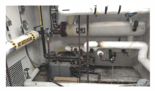
• The existing central heating and ventilating unit for the high school has exceeded its life expectancy and should be replaced with a new dedicated outdoor air handling unit and 25 new 4-pipe fan coil units. FCUs will be located in the classrooms.
