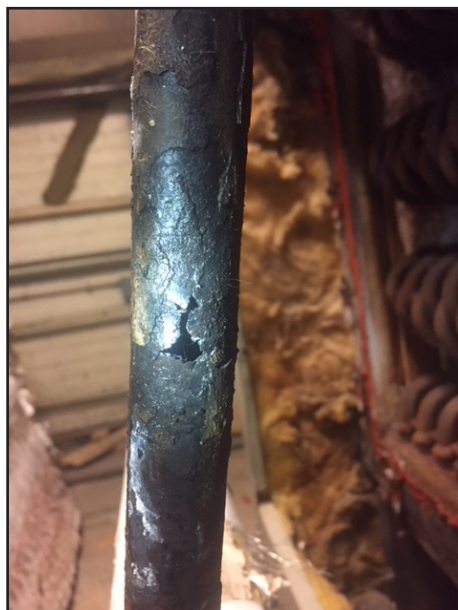
Broken hot water tube
