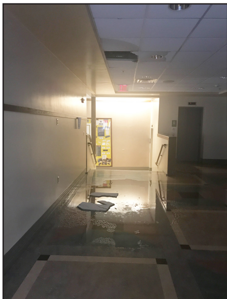
Leak from hot water pump
