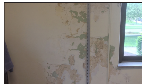
Water damage from roof leak
